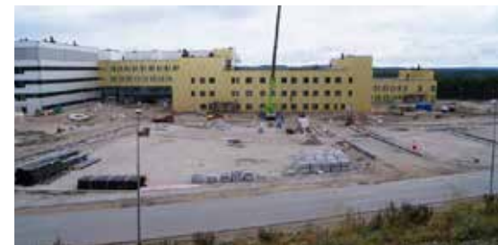
Above: New Østfold Hospital project – model (in Navisworks) and construction works
