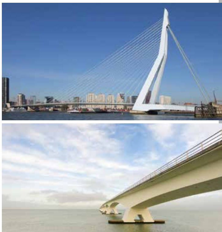
Above: Erasmus bridge over the Nieuwe Maas river; below: Zeeland bridge
